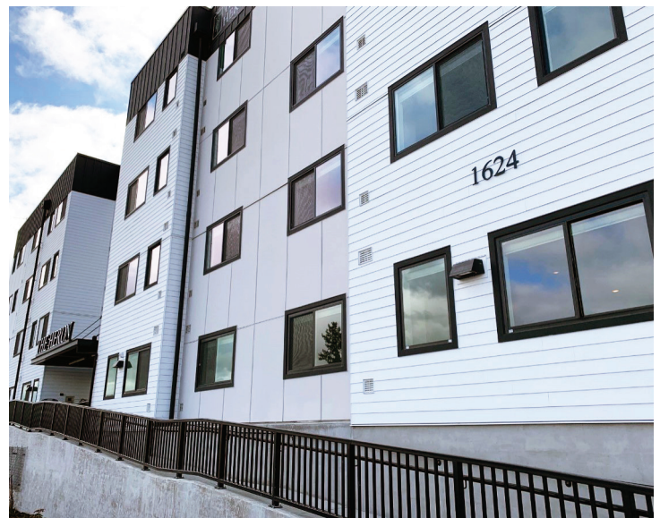
A combination of City of Tacoma and state RCHA funds enabled LIHI to acquire the Heron Apartments in Tacoma
