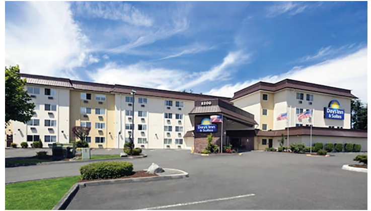
The Lacey Days Inn is being converted into an enhanced shelter
